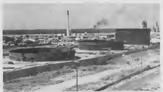
THIS ROW of tanks, each with a capacity of 150,000 barrels, was part of a 1957 tank construction project. Six were built.
